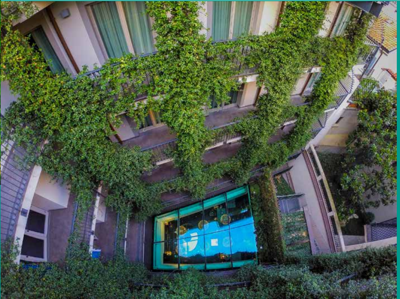
Vertical garden at the courtyard. © Hotel Milano Scala, (Hanna, 2018)
